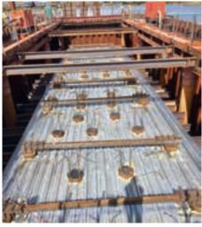
Preparation of concrete slab within cofferdam
