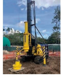
CD-29 rig used to install the H-piles
