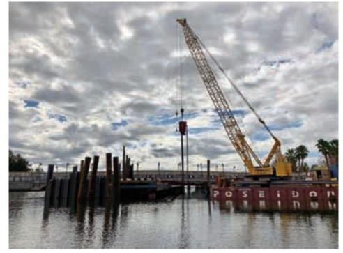
Installation of pipe piles on Hourglass Lake
